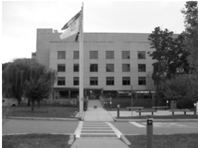
Rockland County Courthouse New City, NY
